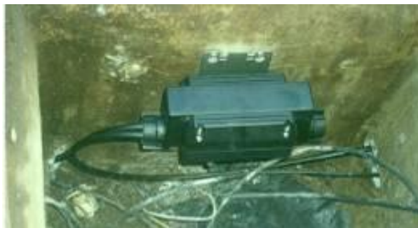
Figure 13: Point de branchement, exemple Nexans 0.2
